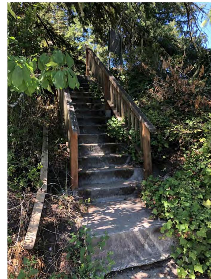
2 EAST BEACH ACCESS STAIRCASE
