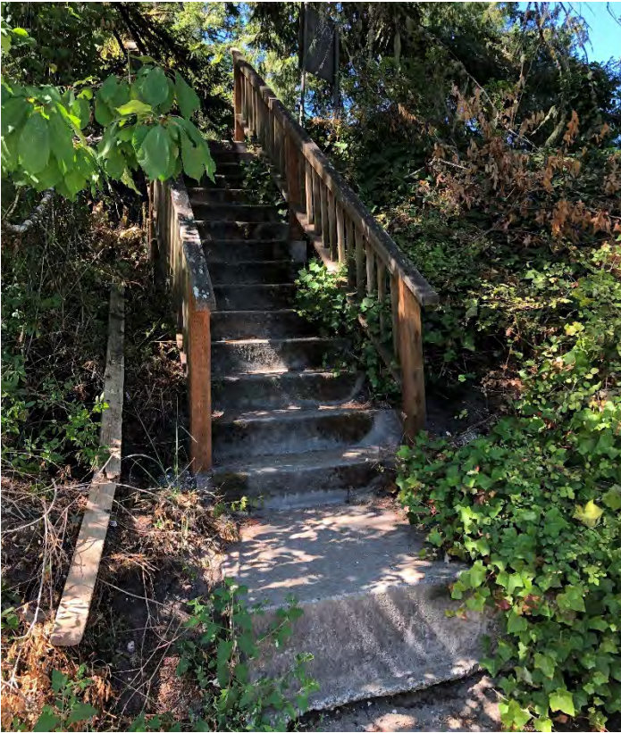
Photograph #7. Eastern Beach Access Staircase (Concrete with Wood Railing)
