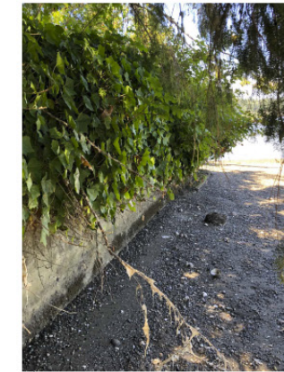
4 CONCRETE BULKHEAD WALL
