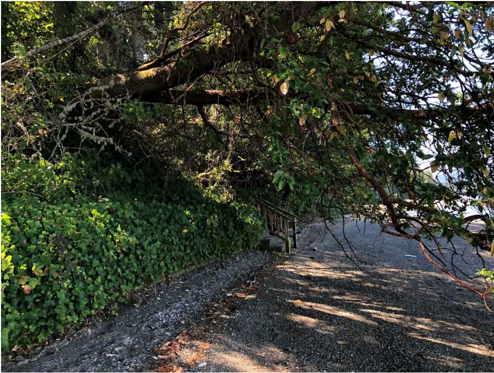
Photograph #-11. Concrete Bulkhead (under overlying vegetation) At Western Facing Shoreline
