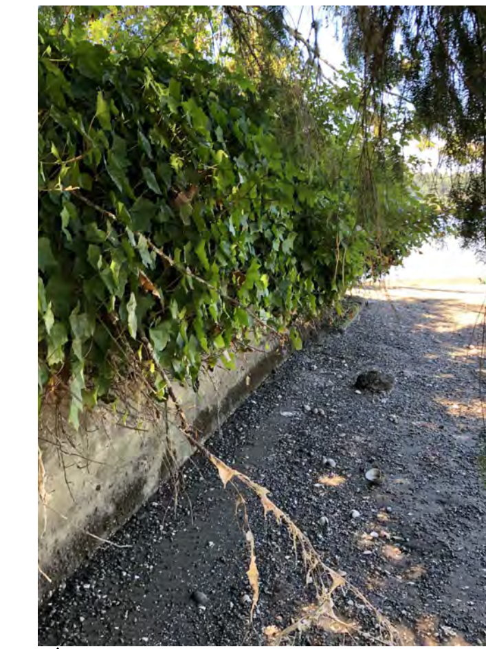
4 CONCRETE BULKHEAD WALL
