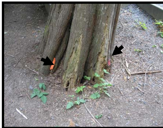
Photo D. View of decay at ground line – between arrows. Nearly 50% of root collar is decayed (WFCI 7/31/08).
